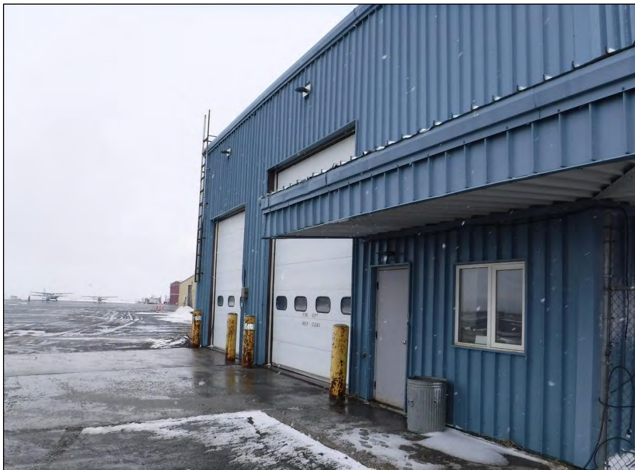
Figure 5-14 Snow Removal Equipment Building
