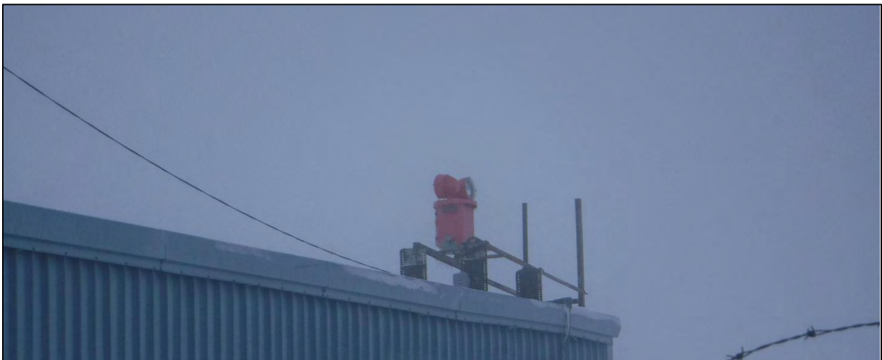
Figure 1-8 Airport beacon located on top of the Snow Removal Equipment Building
